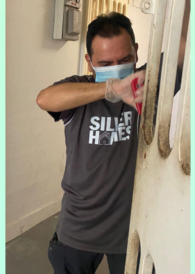
Scraping off old paints
